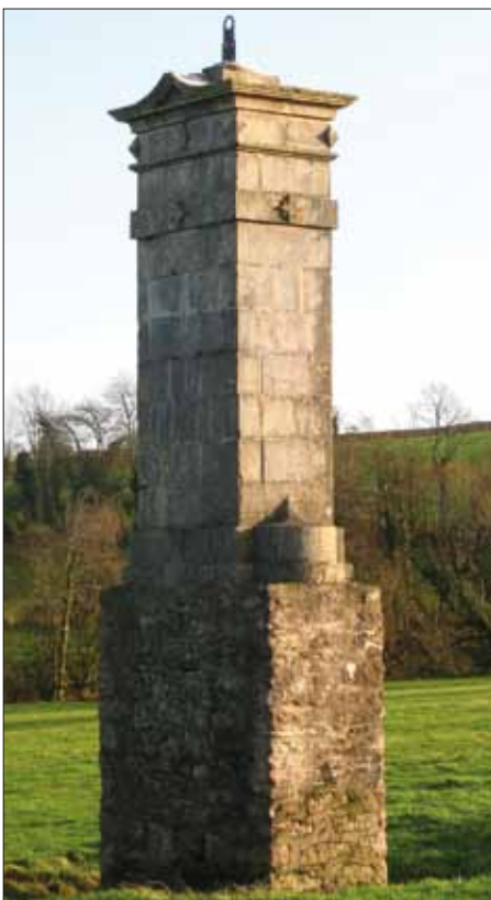
6 The southern meridian mark for the transit instrument at Ballyheridan from the northwest. The stone base and the metal fiducial mark on top were renovated in 1999.
