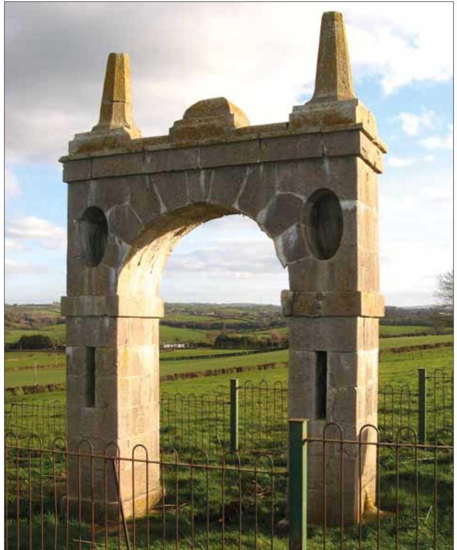
1 The meridian mark at Tullyard for the transit instrument from the northwest. Note the elliptical holes (subsequently blocked) which formed the first stage of alignment and the vertical slits for the second stage. Metal discs mounted on the pinnacles on the top of the arch provided the third stage.
